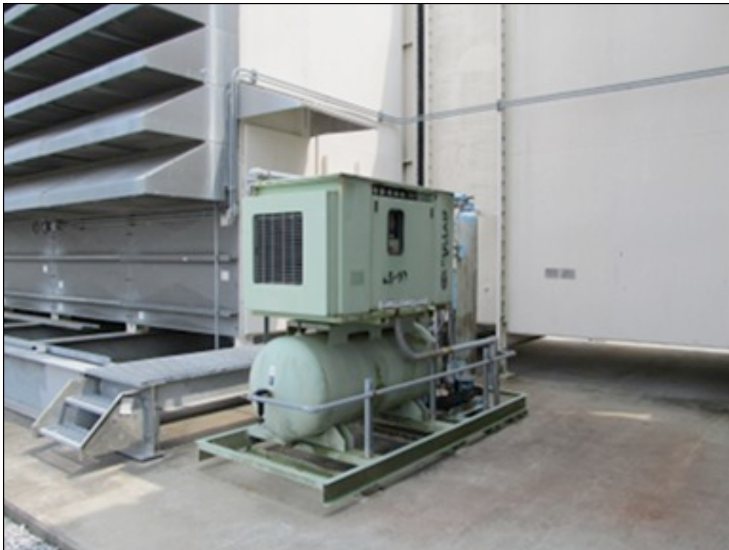
Figure 3 – Pulse Compressor Skid
