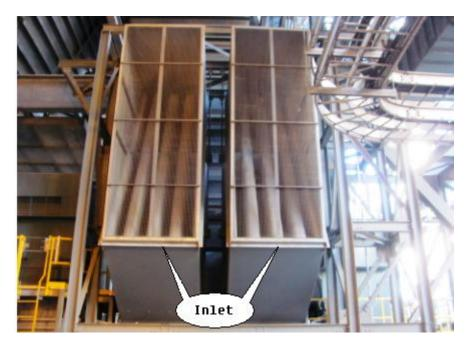
8.2.17 INSPECT drive side variable inlet vane assembly for 360 degree clearance and for damaged vanes and loose or missing hardware.
