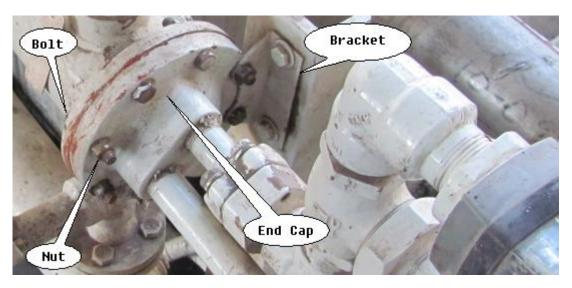
8.4.8 With heat exchanger is supported by sling, REMOVE two nuts and two bolts securing heat exchanger end cap to bracket. PLACE nuts and bolts in zip-lock bag <u>AND</u> LABEL bag.
