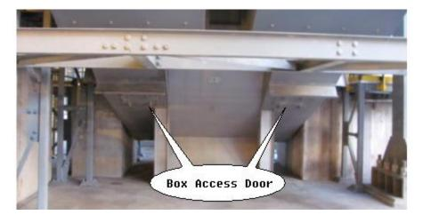
8.2.4 INSPECT box access doors for erosion, corrosion, leakage, looseness, and proper seal.
