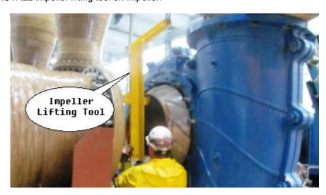
☐ 8.2.38 Using crane, RETRACT impeller from pump casing.
