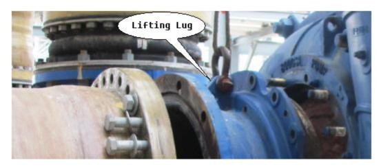
Using crane, REMOVE suction cover from pump <u>AND</u> SET suction cover aside. REMOVE rigging from suction cover.
