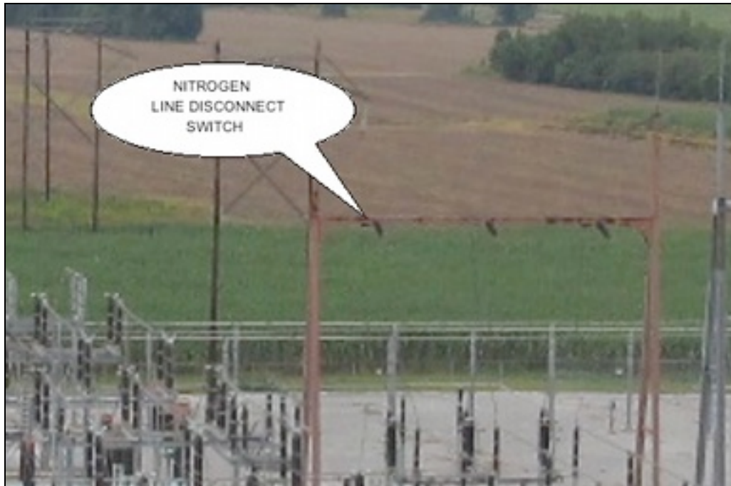
Figure 5 – Nitrogen Line Disconnect Switch
