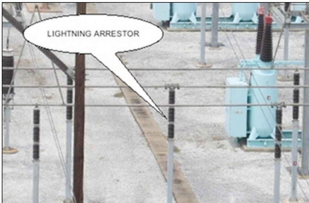
Figure 6 – Lightning Arrester
